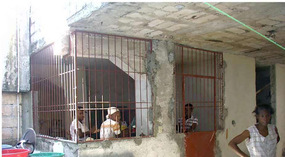
New enclosed kitchen at Kingdom Kids Orphanage. One of many 2007 improvements.
