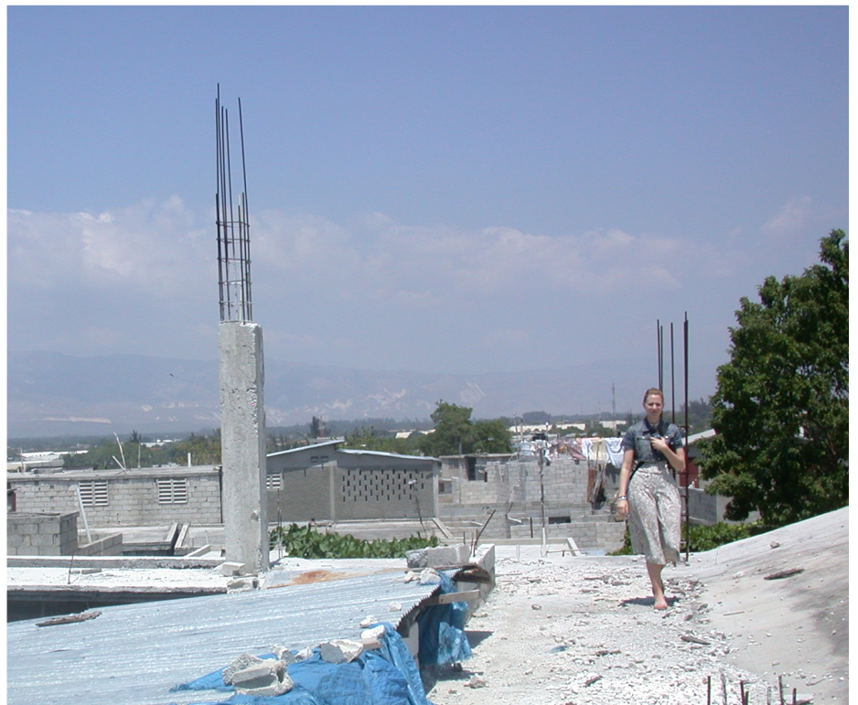
New board member Kristin Scott takes a stroll on the roof of CJRA
